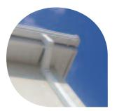
Rainwater refers to the gutters and downpipe system, applied after the fascia and soffit, to channel rain to the underground drainage outlets.
